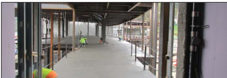
Elevated walkway between library and classroom building concrete pour
