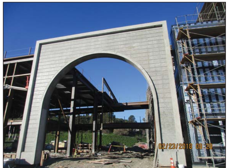
Concrete Archway - Forming Removed and Elevated Walkway Behind
