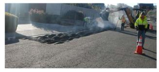
**Description:** Based on the most current P-TAP report various segments will be recommended for slurry seal treatment. A slurry seal functions as a topcoat to existing asphalt pavement to preserve and protect the pavement. It is best suited for pavements with mild to moderate damage, such as narrow cracks, but not for severe damage such as potholes.
