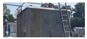
**Description:** In-kind replacement of a 4,000 gallon diesel storage tank used to supply fuel to standby generators and City vehicles. The existing tank is compromised.
