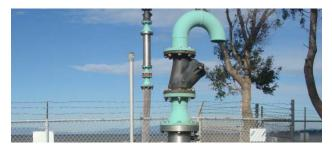
**Description:** Effluent pumping capacity of the treatment plant is limited by the capacity of the pipe size at the effluent outfall in Rodeo. Increasing the pipe size at the Effluent Outfall Eductor Station will increase the wet weather effluent pumping capacity and increase the lifespan of the effluent pipe by reducing the pressure in the line during storm events. Project requires coordination with Rodeo.
