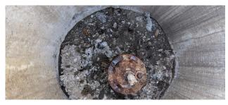
**Description:** There are four air relief valves at various locations on the WPCP Effluent Pipeline between the WPCP and the Rodeo treated water discharge point. This project includes removal and replacement of the pipe saddle, short pipe section, isolation valve, and air relief valve.
