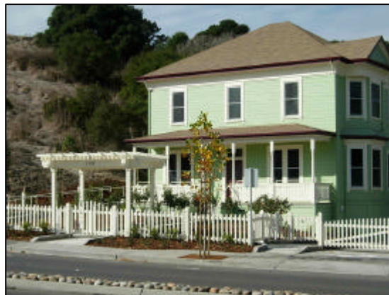
Relocated Faria House
